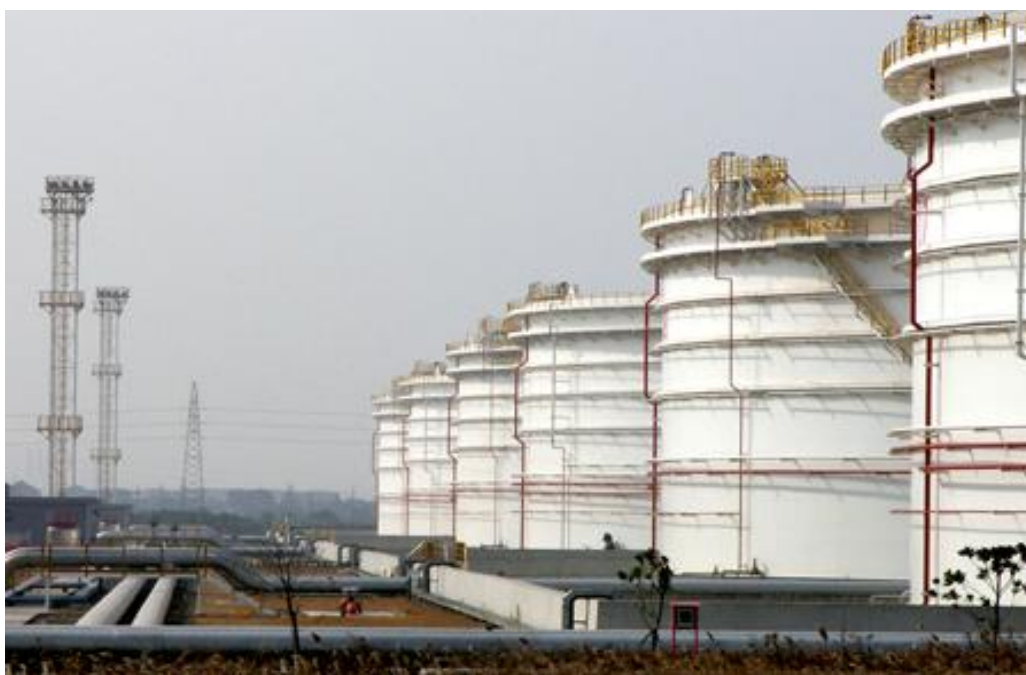
A strategic crude oil reserve base in Ningbo, Zhejiang province
